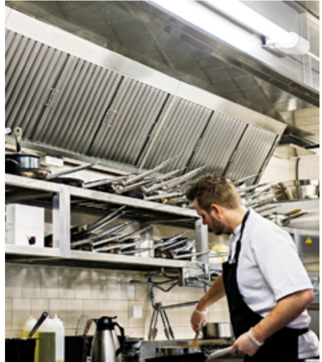
The kitchen hood sucks in the greasy and hot air from the cooking. The air is then continuously treated inside the ducts with ozone.
