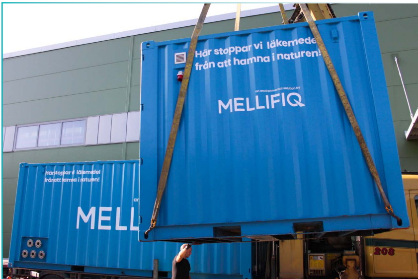
Exterior of the containerized systems with ozonation, adsorption and nanofiltration.
