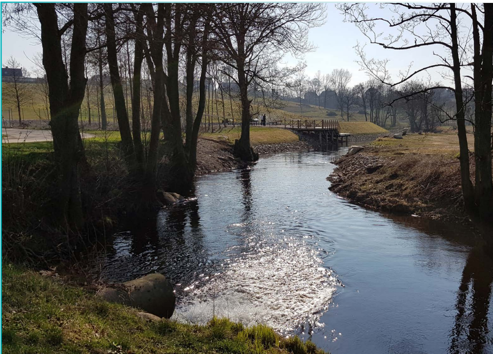
Image from Klippan wastewater treatment plant.
