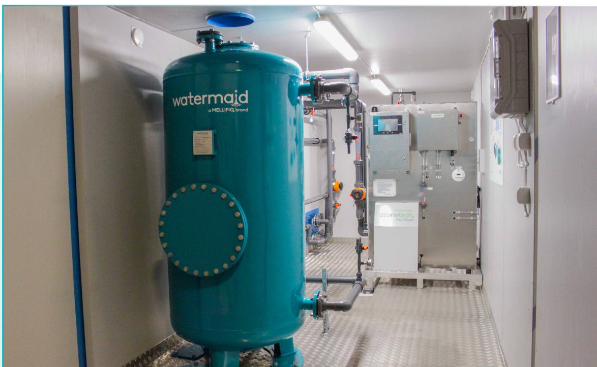
Pilot treatment containerized system with the Mellifiq O-GAC™ process.
