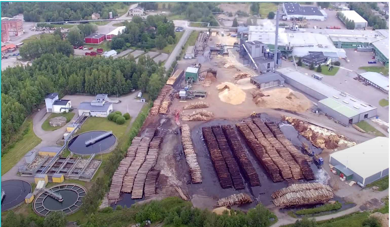
Image from the Pitkäniemi wastewater treatment plant.
