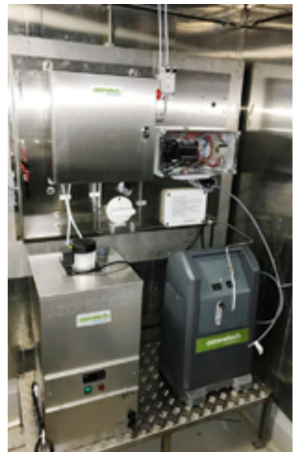
The RENA system to the right includes ozone generator, oxygen-generator, closed cooling system, ozone sensor and the O3Eye control unit.
